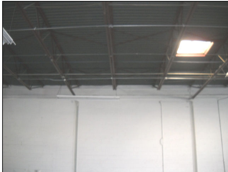
View of structural components and build methodology.
