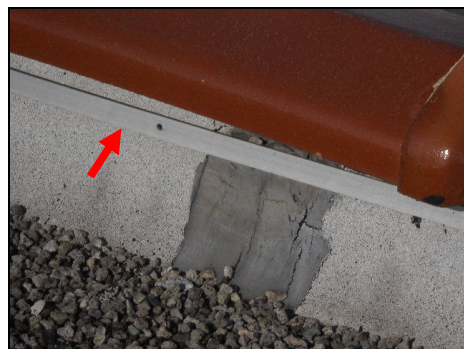
Loose support bands and coping observed at multiple areas.
