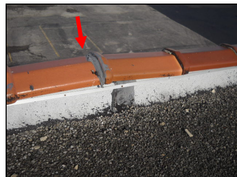
Loose support bands and coping observed at multiple areas.
