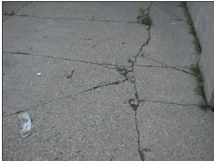
General condition of concrete serving the truck well.
