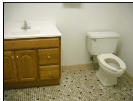
Representative view of bathroom fixtures.
