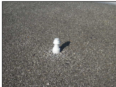
Roof well vented.
