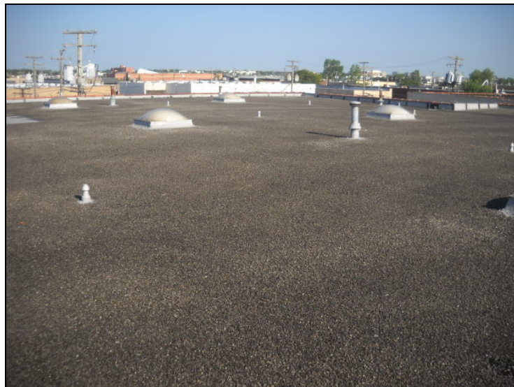
View of roof surface.
