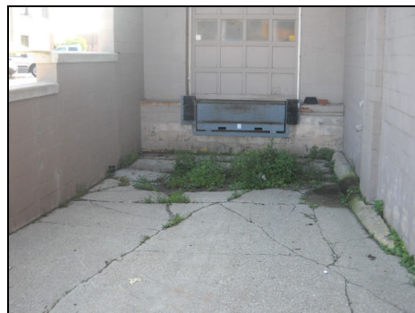
View of truck well.
