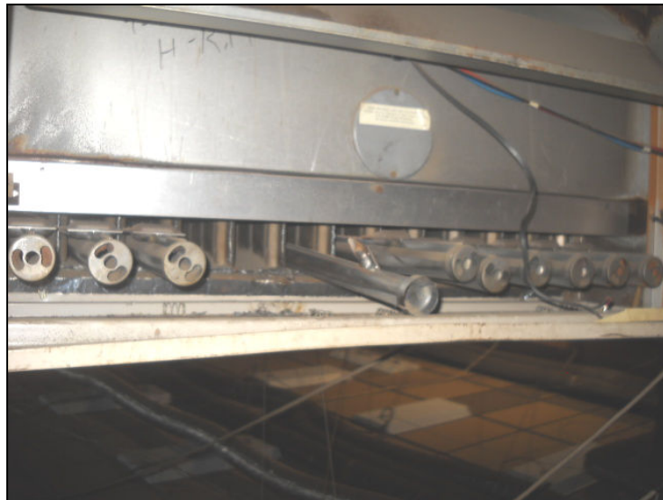
Unitary heating system partially dismantled.
