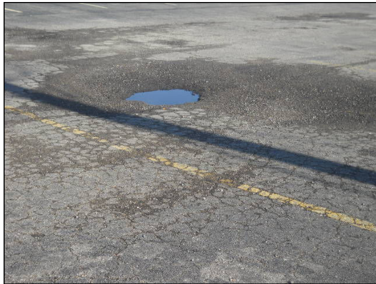
General condition of driveway asphalt.
